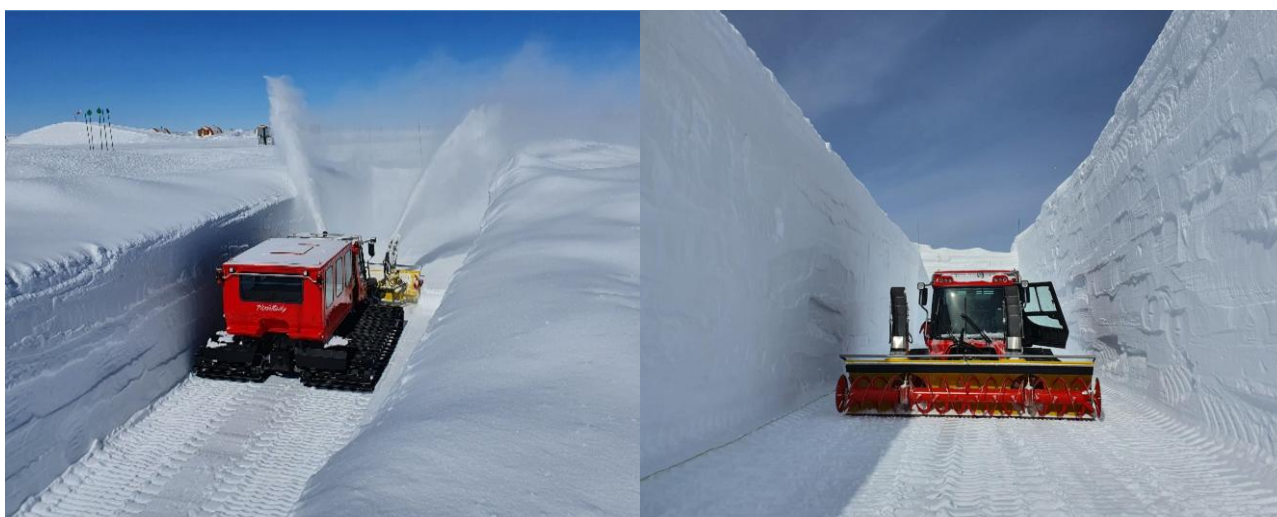
Figure 1 – Excavation work for the construction of the Ice Memory storage cave. A snow trench was dug to a 10 meter depth with a snow blower. Credit: Rocco Ascione, ENEA-UTA, Italy.
