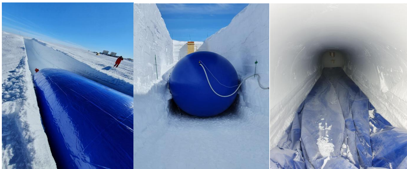
Figure 2 – Building the snow arch of Ice Memory storage cave. A 35-m long balloon is inserted in the snow trench, inflated, and snow is blown back on top of it. After deflating the balloon, the cave has a snow roof modifying slowly over time, without need of any construction material and providing optimal storage conditions at a constant -52^{\circ}\text{C} temperature. Source: Rocco Ascione, ENEA-UTA, Italy.
